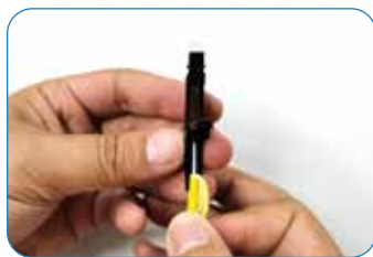
2.9 Put the cable into the boot
